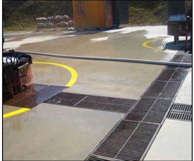
**Fig 11:** Channels through which water flows from fire fighting.
