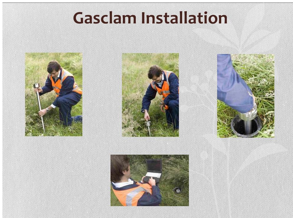
Figure 2: Process of Gasclam installation
