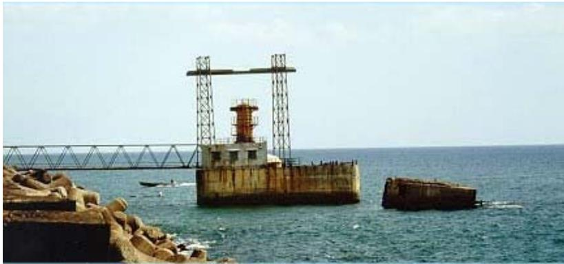
FIG 2. THE OWC PROTOTYPE DEVELOPED AT THE IIT
